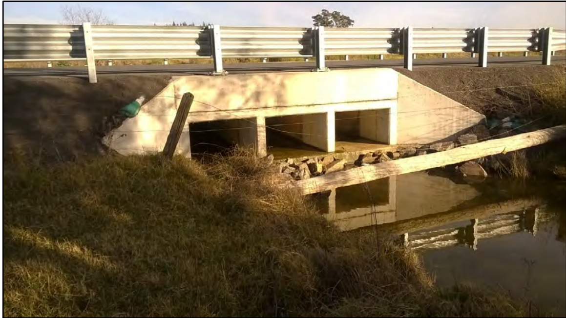
Figure 5: Existing culvert under Wine Country Drive
